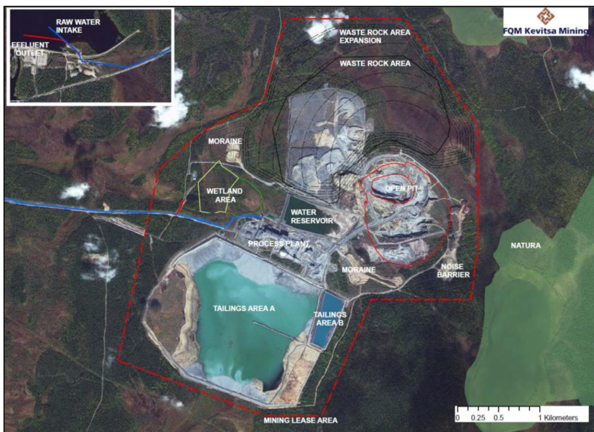
Figure 16-1 Plan view of the Kevitsa mine site, illustrating the pits, dumps and tailings facilities.
